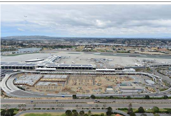
Figure 7: Terminal 2 Parking Plaza (Source: San Diego International Airport Authority)
